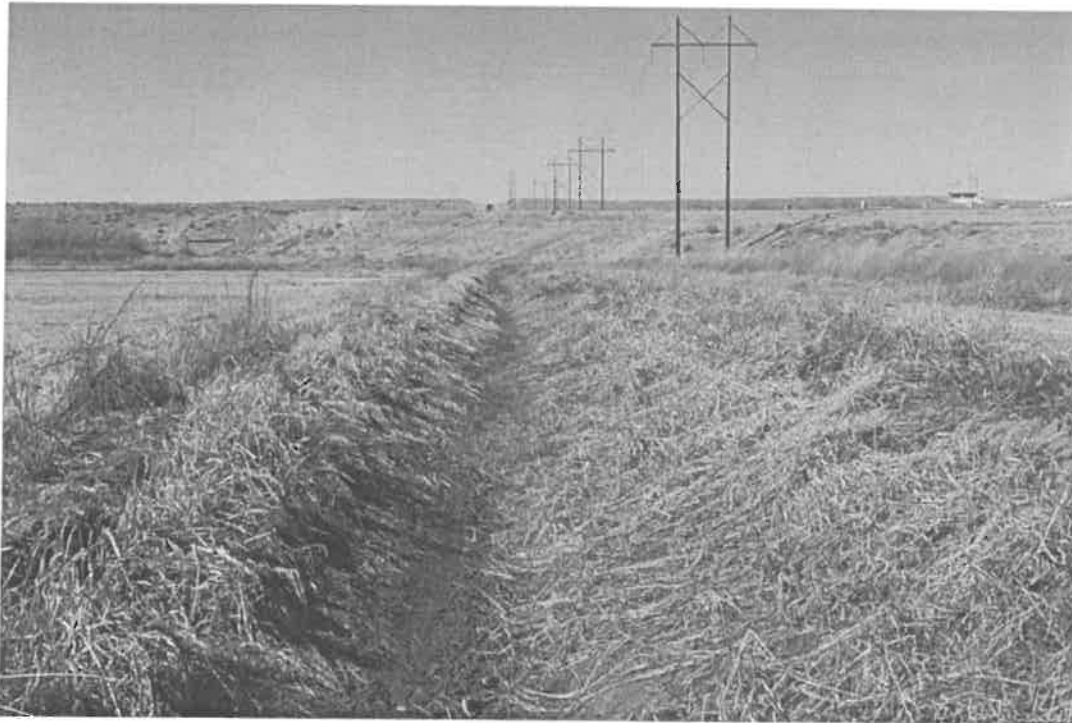
Figure 7. The earthen Ditch B, running west along the power line.
