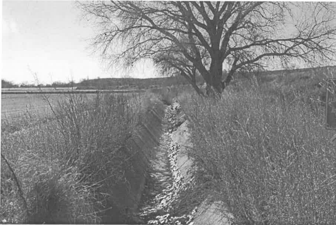
Figure 8. Looking south down concrete-lined Ditch C.
